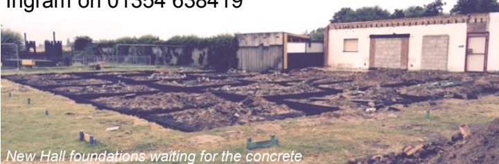
New Hall foundations waiting for the concrete
