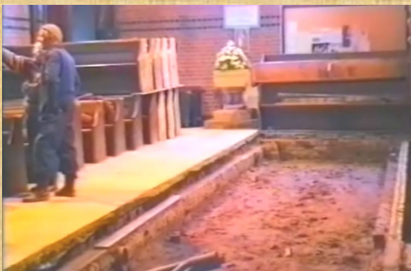
with the rotten floor removed
