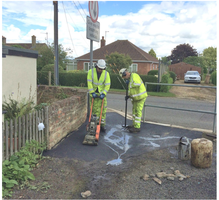
Ricky and Daniel use a vibrating plate to ensure a smooth change of level
